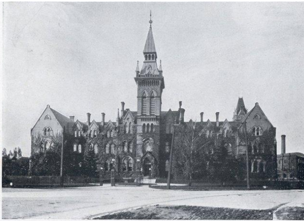
KNOX COLLEGE (PRESBYTERIAN) Situated at Spadina Avenue Crescent, with street cars looping it on either side. Beautiful with vines in the summer and fall. Plain and stern of architecture, typical perhaps of its ancestry. Dr. Owen
