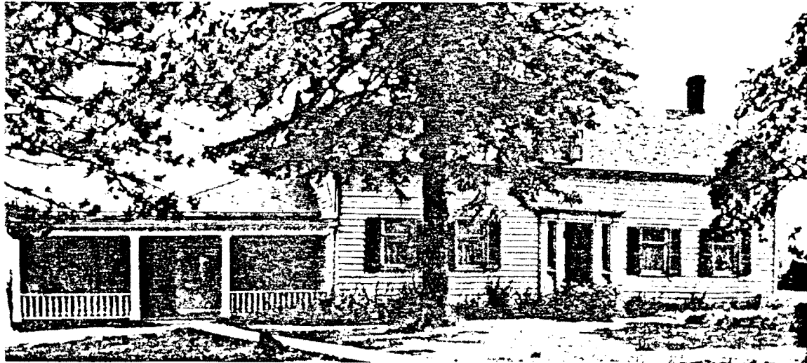
A view of the front of the Noxon/Guernsey House taken in 1925, the doorcase intact and the dormer, curiously off-centre, in place, but the windows already showing a c. 1900 improvement: the bar across the shutters suggests the original arrangement of a sash of twelve panes above one of eight. (From the Meredith Collection: courtesy Public Archives Canada)
