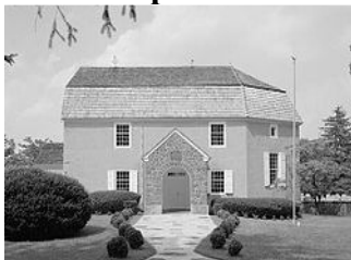
Old Trappe Church, built 1743
