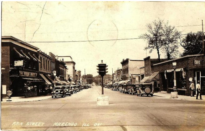
1910 approx Main Street in Marengo, Ill
